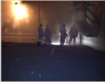
Internal coating of Degassing tank Qatif GOSP#2
