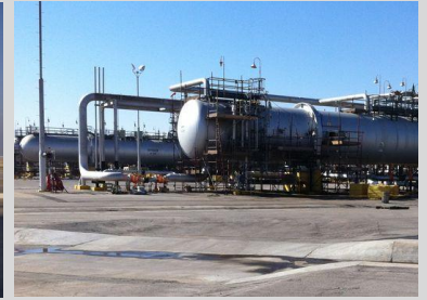
Recoat of all tanks and vessels full shutdown - Aindar GOSP#1
