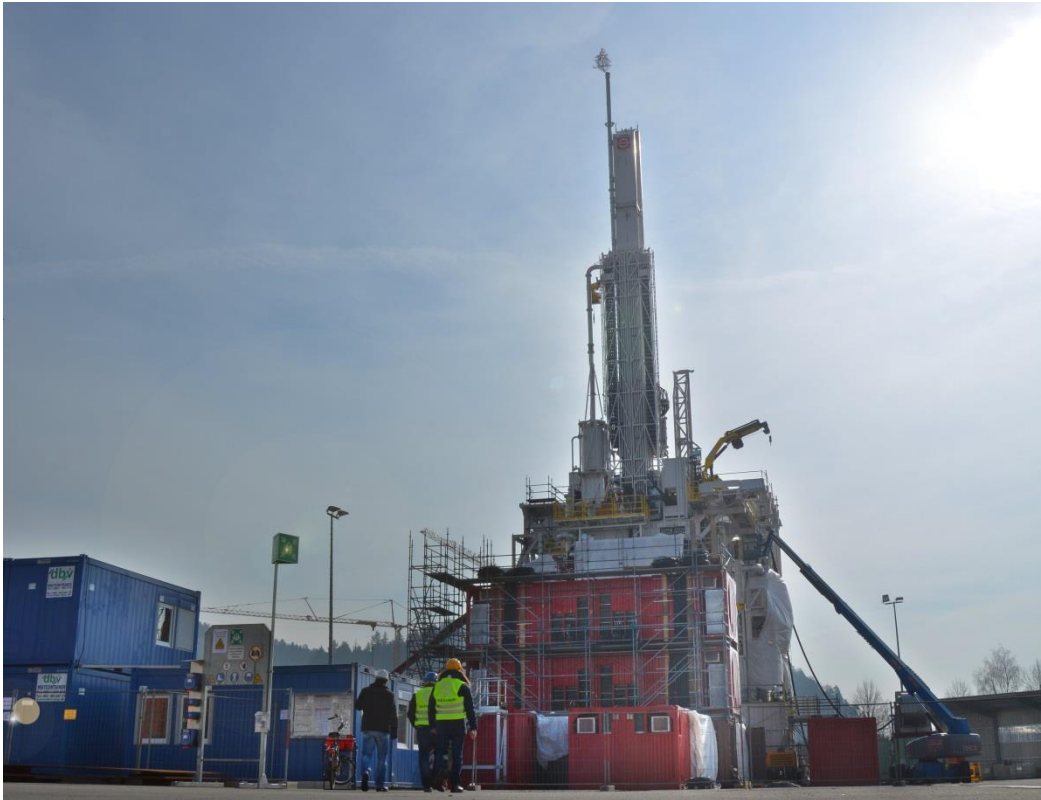
Fig. 1: It's not a UFO, it's the VDD 400.2 offshore deep drilling rig from MAX STREICHER GmbH & Co. KG. in Deggendorf, Lower Bavaria. (Photo: Jacob)
