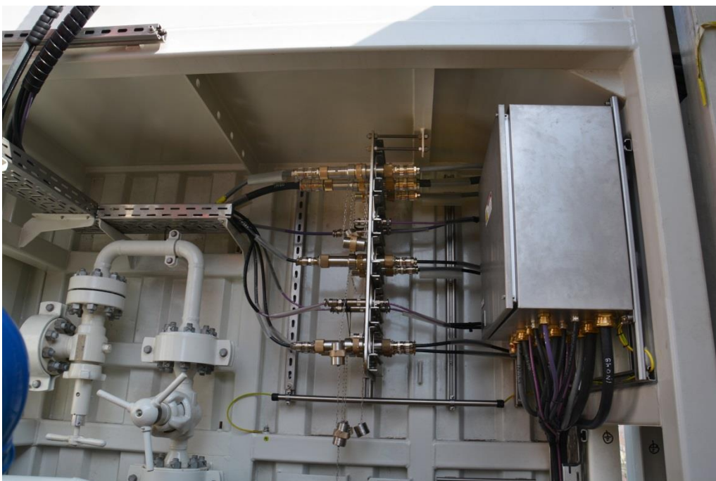
Fig. 3: HAWKE connectors (l) and HAWKE cable glands (r) in use – created for tough and potentially explosive environments. (Photo: Jacob)
