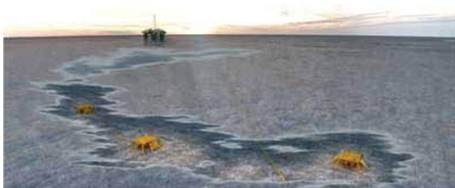
Three subsea templates tieback to Gjøj platform.
