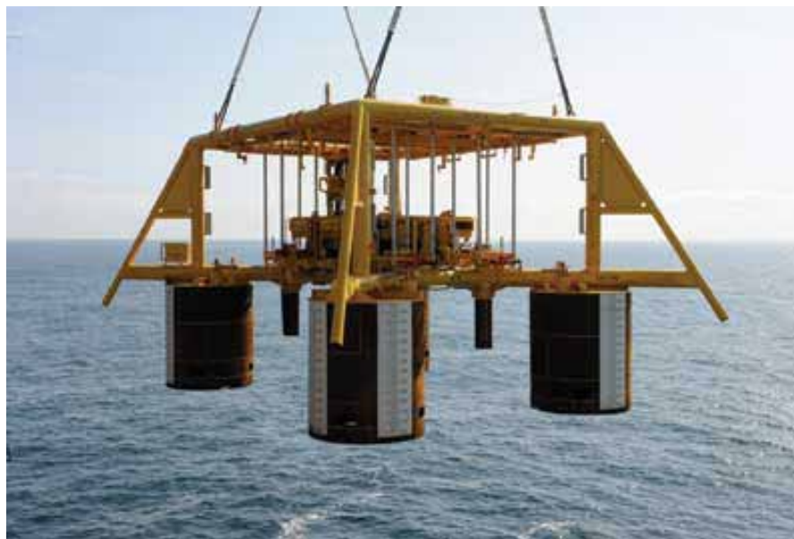
Subsea template being installed from crane vessel Thialf. Photo: AndreOsmundsen/Statoil.
